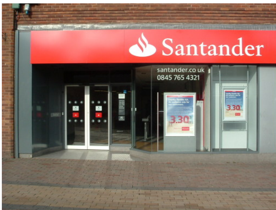
Picture 5 Entrance doors contrasted from frame ensures entrance is easily identifiable. Appropriate use of manifestation and level access.
