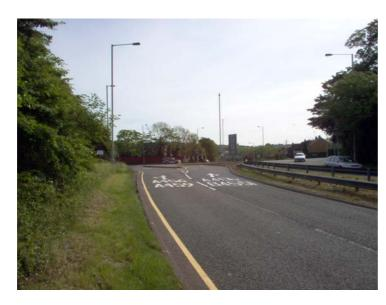
The lack of flare on the approach to the Stop line on the Birmingham bound carriageway restricts capacity here and could be rectified by local widening approaching the roundabout.
