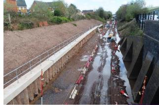
33,000 tons of ballast have been delivered ready for track to begin being installed across the railway corridor this autumn.
