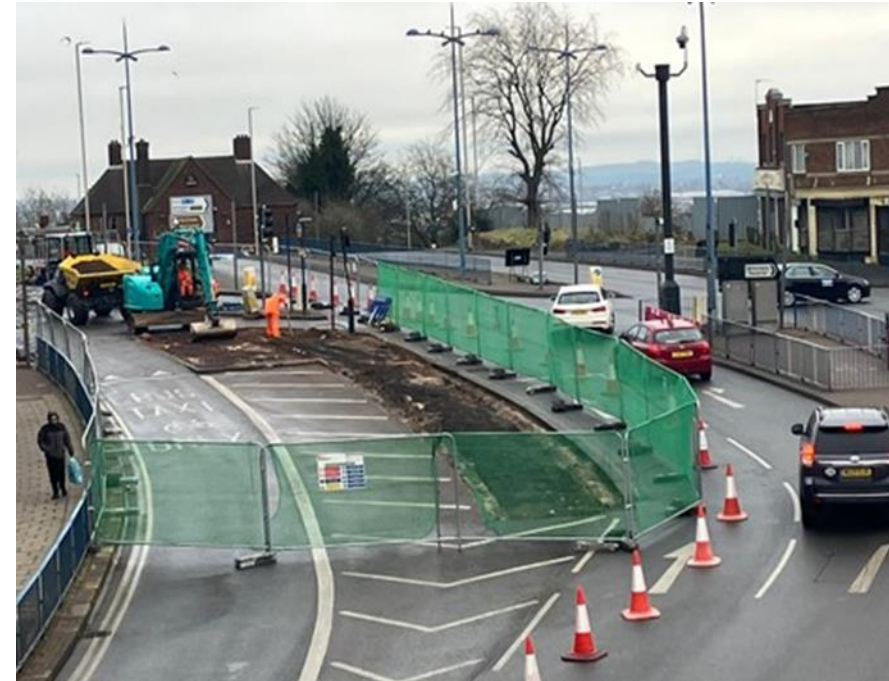
King Street splitter island removal
