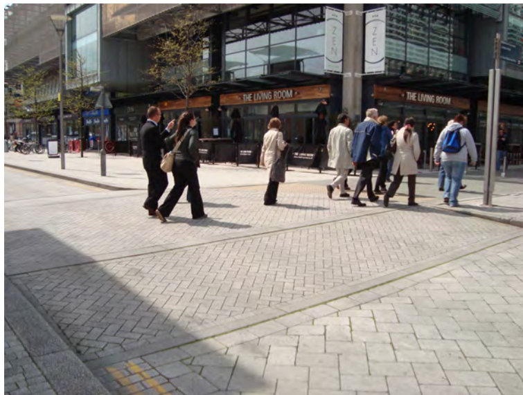
Figure 5.42 Careful choice and combination of paving materials act to provide accessible public routes which are hard wearing and attractive links through a place (Bristol City Centre)
