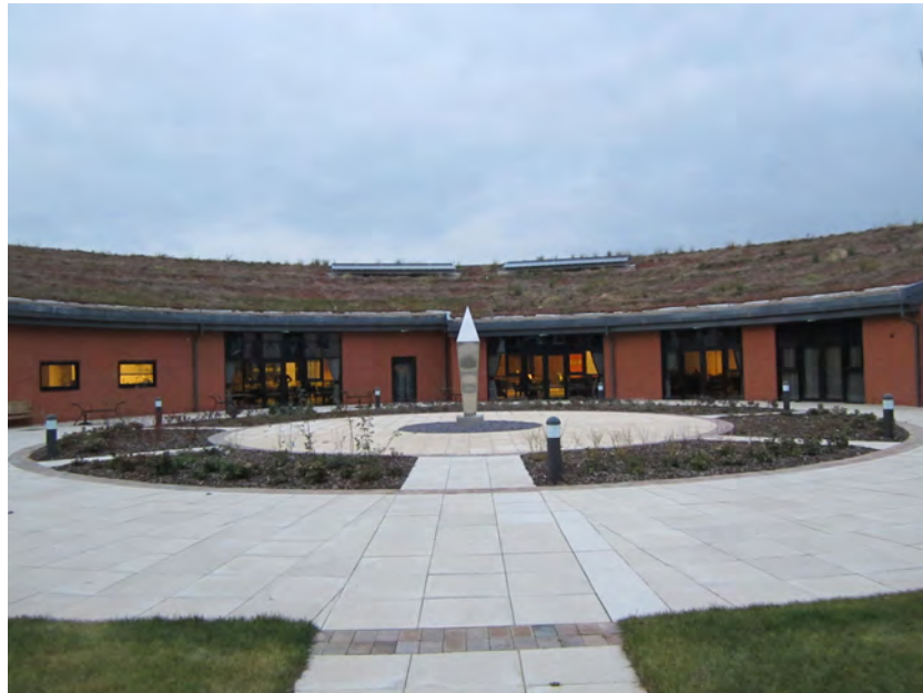
Figure 4.12 Illustration of green roofs used in new housing development (Middlepark Road, Dudley)
