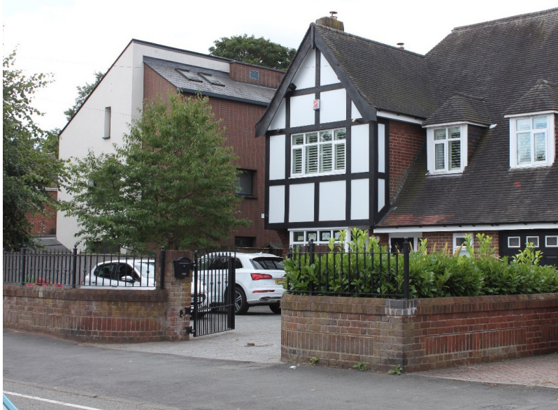
Figure 2 Eco Vicarage, Kingswinford to left of photograph which achieved Code for Sustainable Home Level 6 and Passivhaus accreditation. Note the use of height, roof pitch and materials that take design references from the adjacent house
