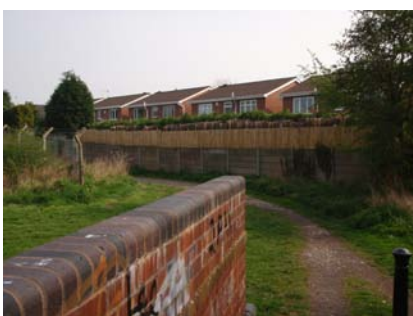
Poor quality public space along the canal towpath
