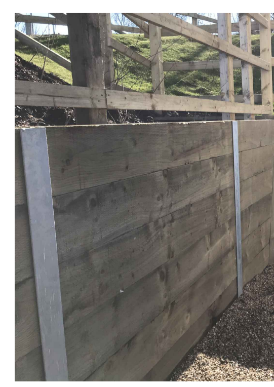
TIMBER SLEEPER WALL WITH STEEL POSTS - TYPICAL IMAGES
