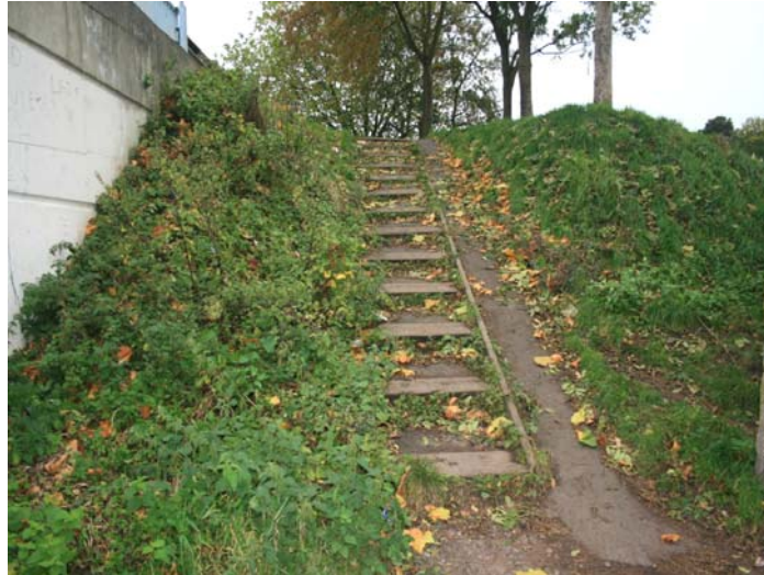
Fig.5 The ramp at Longboat Lane Bridge
