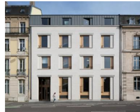
Nos. 31, 32 and 33 Hall Street demolished and replaced with sympathetic new build
