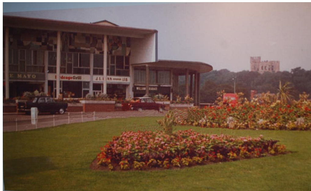
Figure 28 – Photo of the Churchill Precinct c.1970's.
