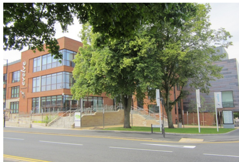
One of the new Dudley College Buildings, Evolve
