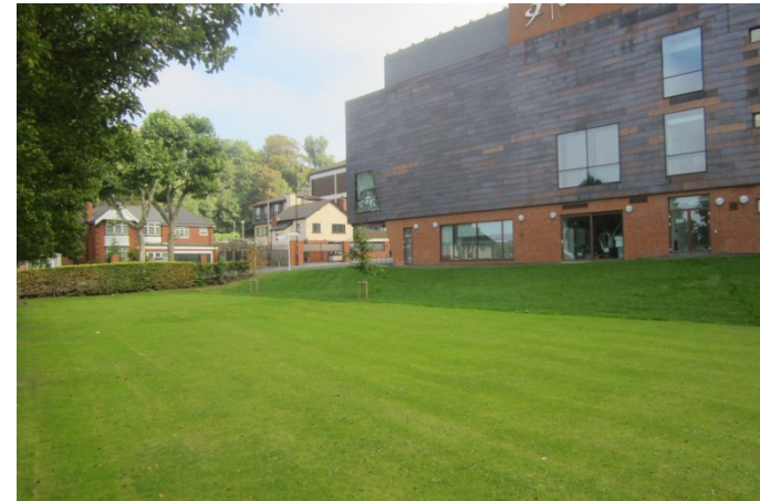
Rear of the Evolve College Building
