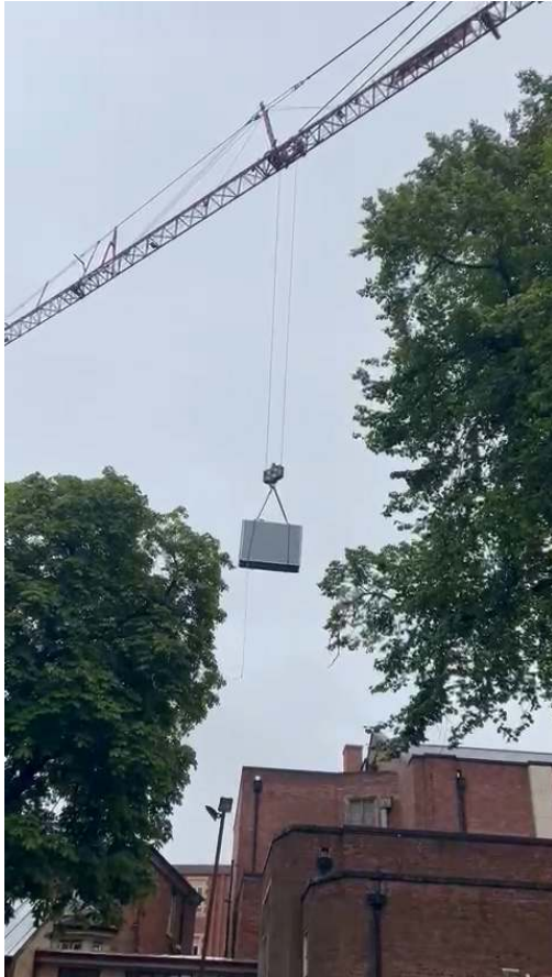
Heat recovery fans being craned into position
