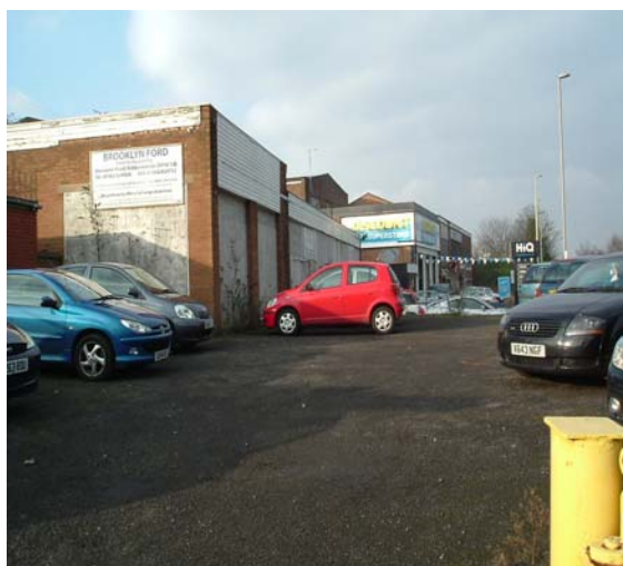
Site E – Northern tip of the Angel Passage site. View taken adjacent to Birmingham Street (A458) looking north-west across car sales uses (some car sales premises now derelict). (Date photograph taken: 25 th January 2010)
