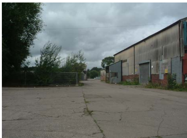
Site D – View of derelict industrial units located between Canal Street and Bradley Road. Former Stourbridge Rolling Mills site. View looking west (Date photograph taken: 25 th August 2009)
