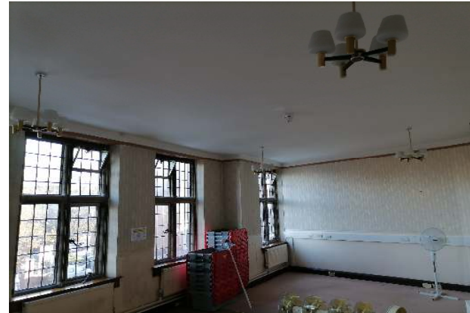
Members Room - before
