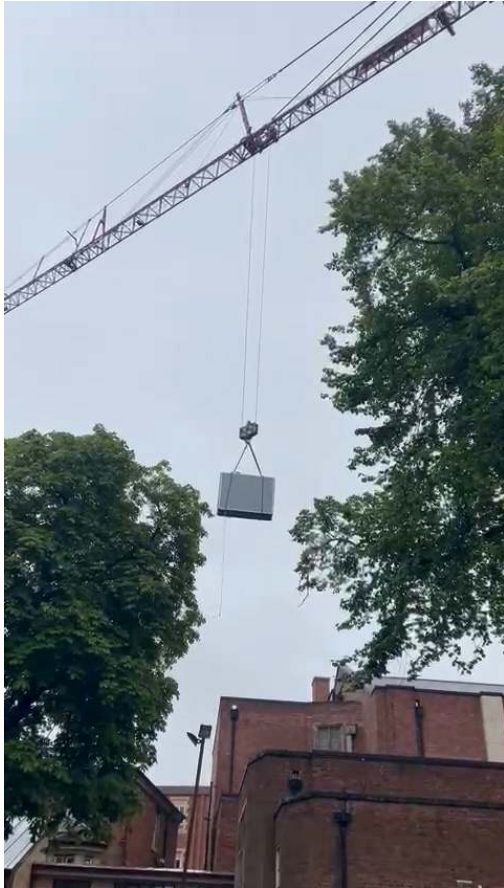
Heat recovery fans being craned into position
