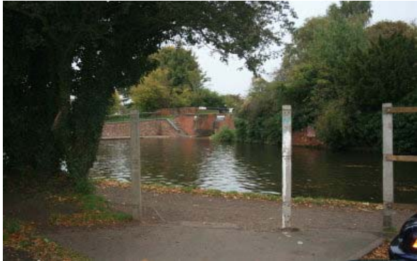
Missing fence posts at the end of Smallshire Way
