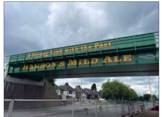
Hanson's Bridge restored to its former glory
