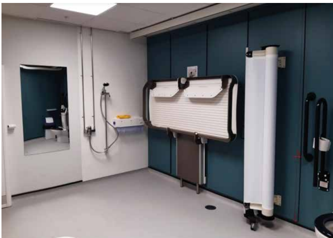
Photograph of the completed toilet
